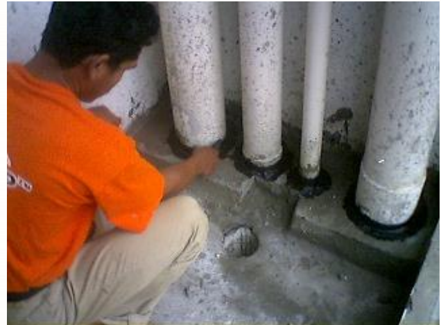
* Typical treatment to down pipe.
